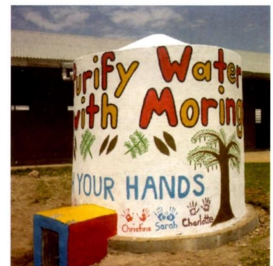
Completed water tank
